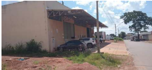
- RUA EVEREST, QD. 64, LOTES 9 A 12 -
