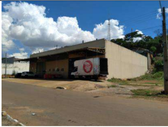
- RUA EVEREST, QD. 64, LOTES 9 A 12 -
